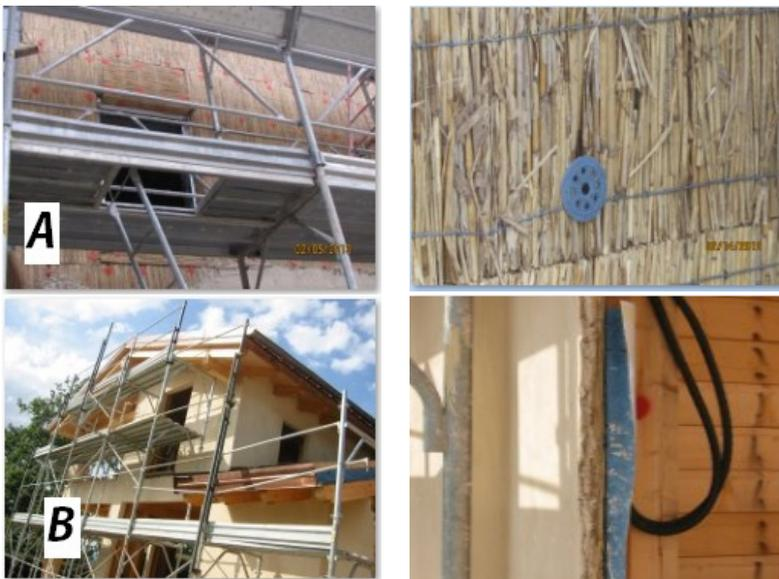
*Fig. 3 – Common reed panels are used as outside insulators in a masonry building at Castelfalfi, Tuscany (a) and in a wooden building on the Trasimeno lake (b) (courtesy of Lincep, S.Savino-Magione, PG, Italy).*
